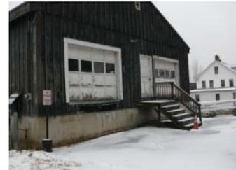
3 Attic louvers are damaged. If building is re-insulated the louvers should be removed and wall patched.
