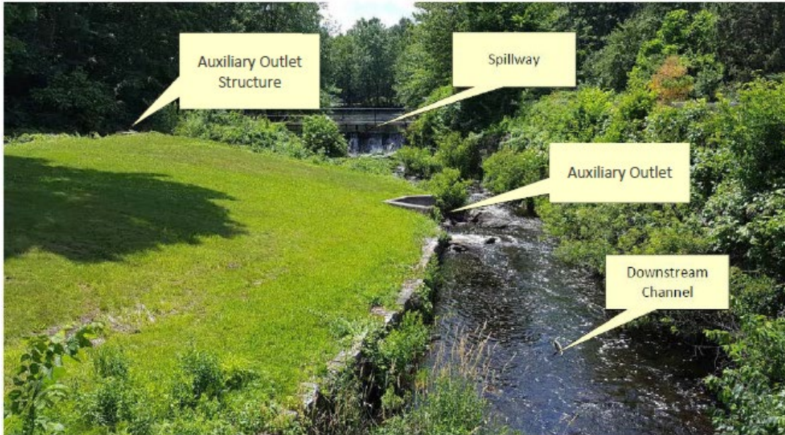
Figure 5: Downstream of Forge Pond Dam and Auxiliary Outlet
