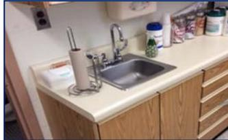
3 Sinks and restroom in Health Clinic are not ADA accessible. Knobs on doors need to be replaced with lever type hardware.
