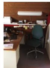
Carpet throughout Second floor need to be replaced. Vinyl tile floor are worn under chairs. Replace with sheet vinyl.
