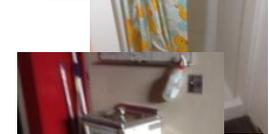
Water cooler is not ADA compliant. Replace with dual height unit.
