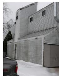
Areas of the aluminum siding are dented or have been partially replaced. The building in total has a shabby appearance and consideration should be given to replacing the siding material. Alternatively, exterior of building should be washed.
